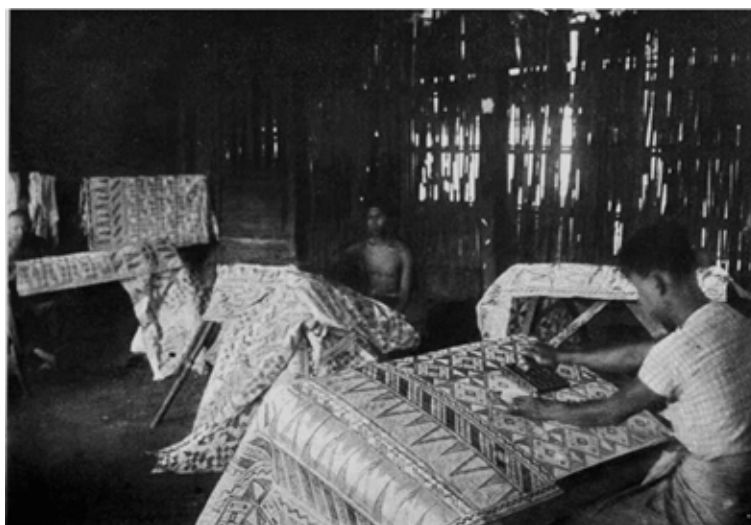
Fig. 6. Batik production with copper stamp technology.
